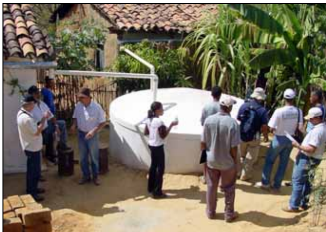
Rooftop catchment system installed for household water supply (above, left) in rural Brazil. Using the AWW bacteriological testing protocol to test residential water supply (above, right).
